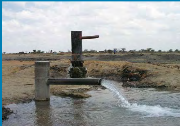
Artesian borehole in central, semi-arid Tanzania
